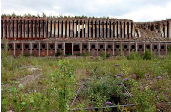
Fig. 2 Remains of the coke plant at Dortmund
