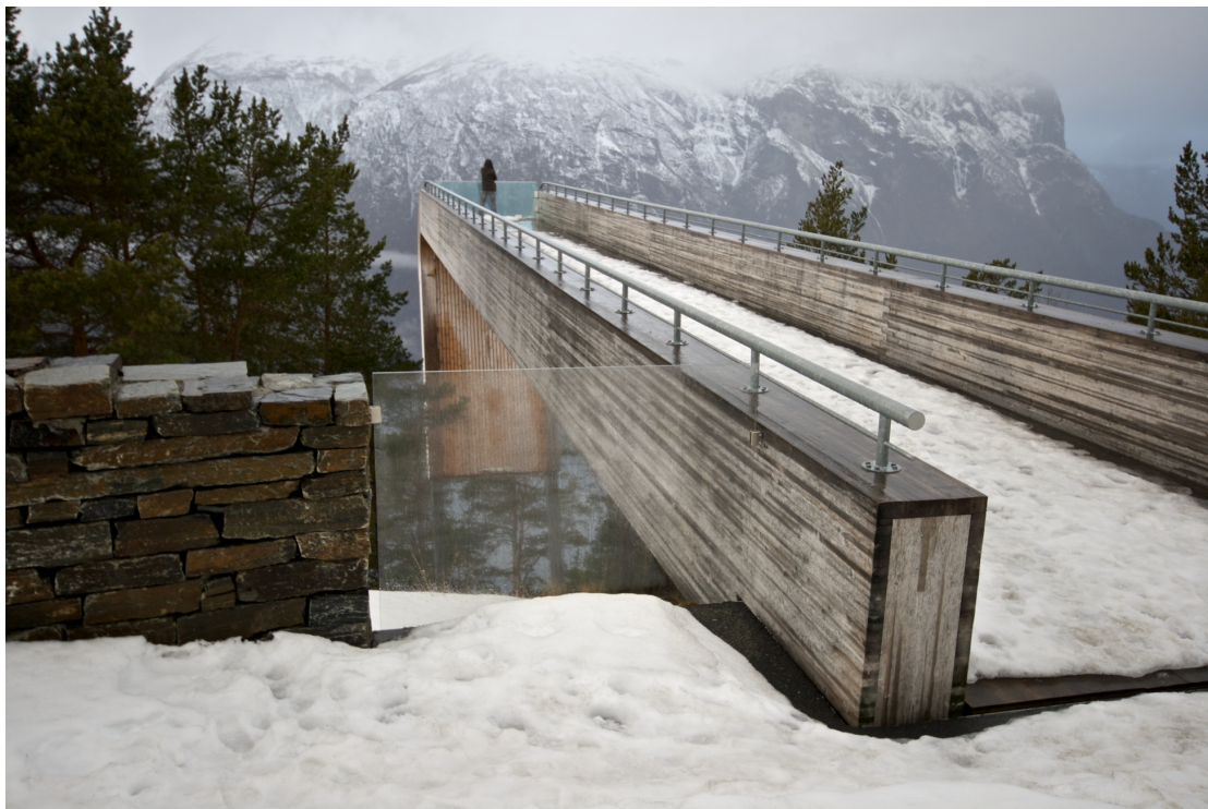
Figure 1: Stegastein platform in March
