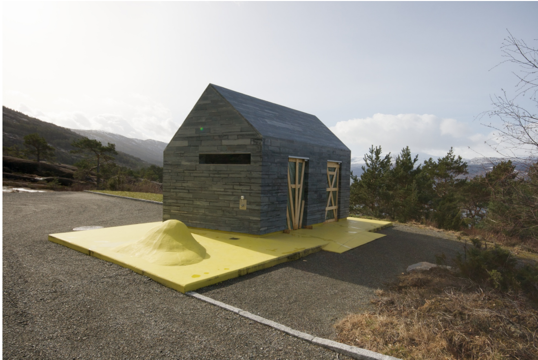
Figure 2: Hereiane toilet building in March
